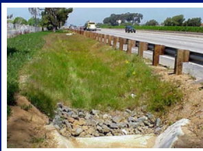
Roadside Vegetated Swale; source: dot.ca.gov
